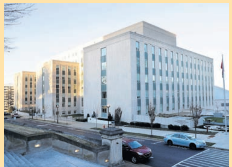
The Cordell Hull State Office Building stands, Jan. 8, 2020, in Nashville, Tenn.
